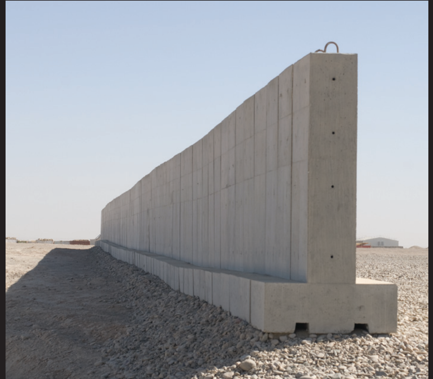
DAVID COTTERRELL, THEATRE (2008). FLIGHT-LINE BLAST-BARRIER, BASTION.
